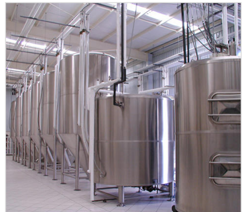
Fermentation tanks made of stainless steel. After the addition of yeast the fermentation process creates the beer's alcohol and carbon dioxide.
