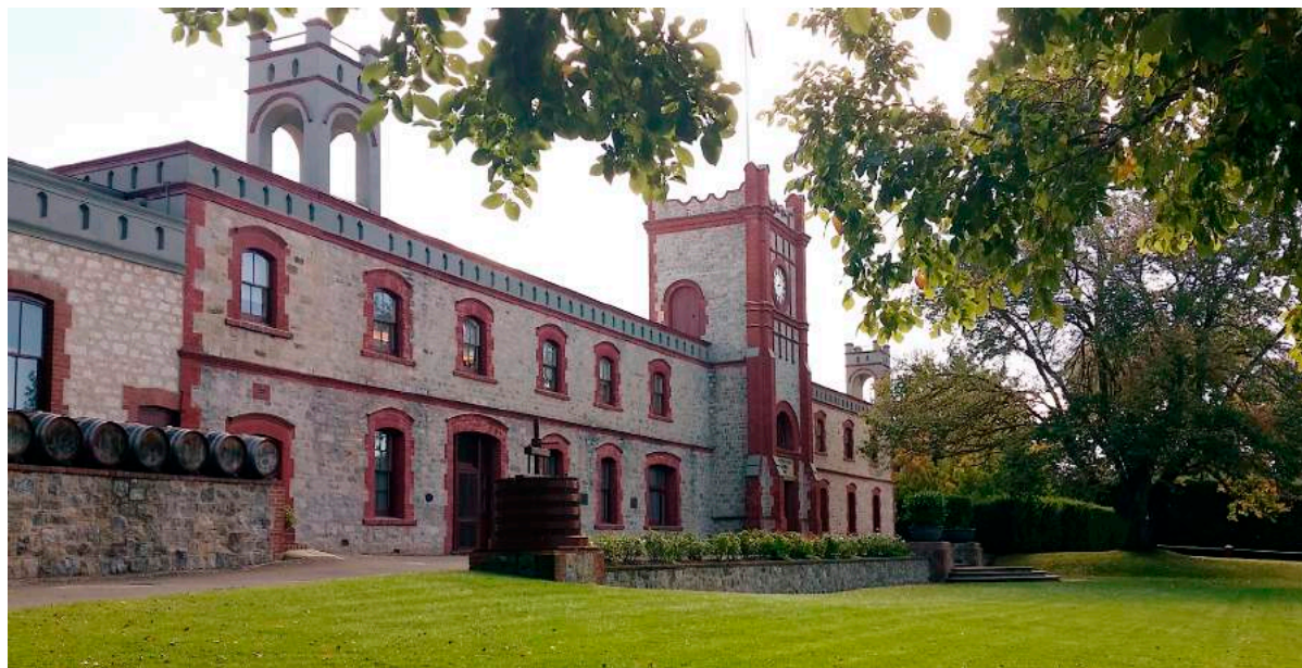
Yalumba winery. The winery is serious about reducing energy costs, and monitors energy consumption continuously.
