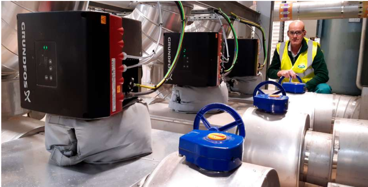
Figure 5: Intelligent control modes ensure secure integration of NKE and NBE standard pumps and end suction pumps, for example, with TPE inline pumps in cooling water circuits.
